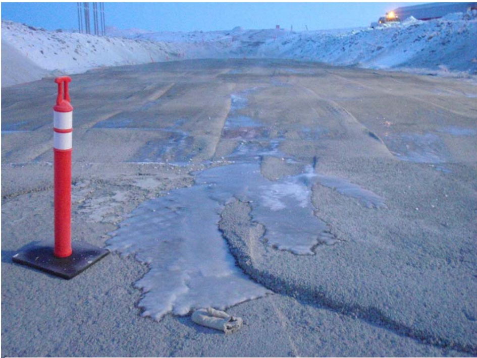
Photo 2: Ice formed from water bleeding out of the material placed 2012/02/01 nightshift. Photo looking north east along key trench. Note that this was the most notable area like this.
